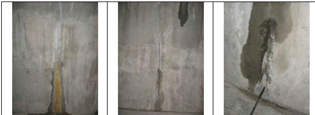
Identify the leaking crack and chisel it out as per Application Instruction 5.11 – Waterproofing Cracks, Holes & Joints
