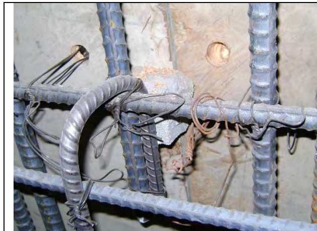
Remove excess tie wires
