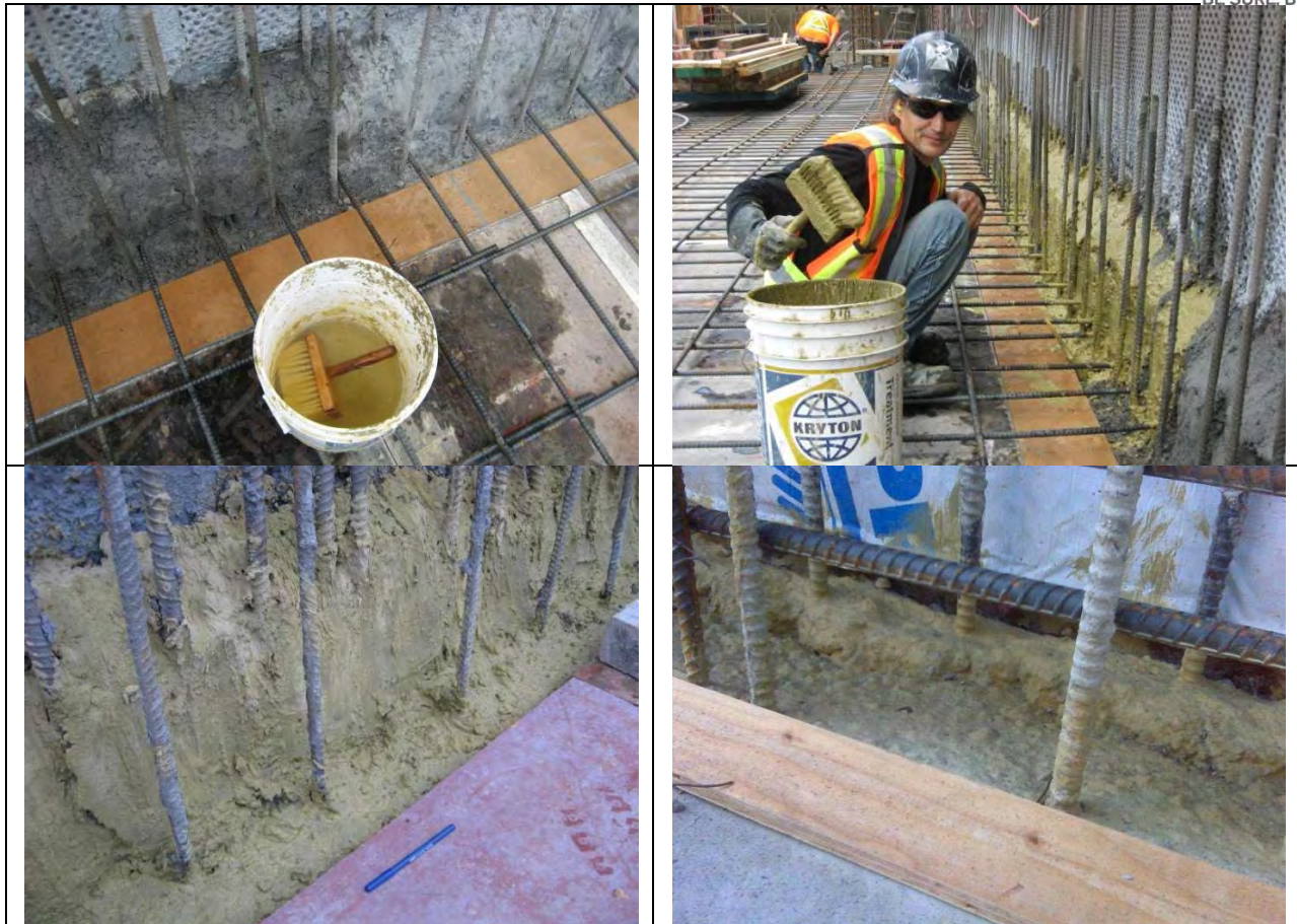
Installation of Kryton Waterstop Treatment. Refer to Application Instruction 4.12 – Waterproofing Horizontal and Vertical Construction Joints (External Method)
