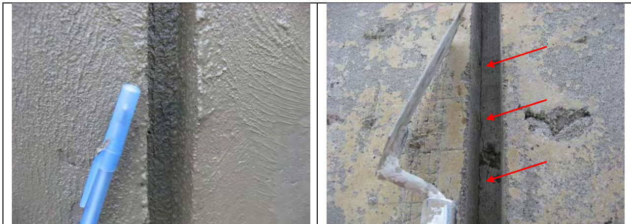
Typical control joint reveal
