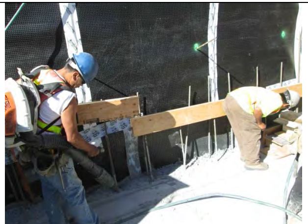
Remove all debris from the joint
