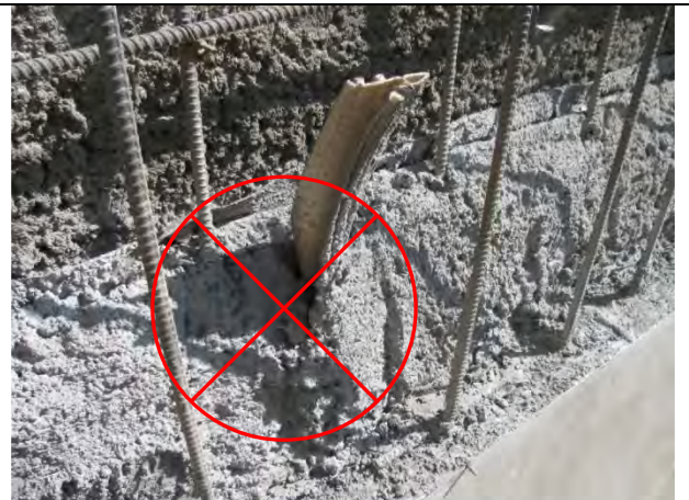
Folds or twists at the top will interfere with slab placement
