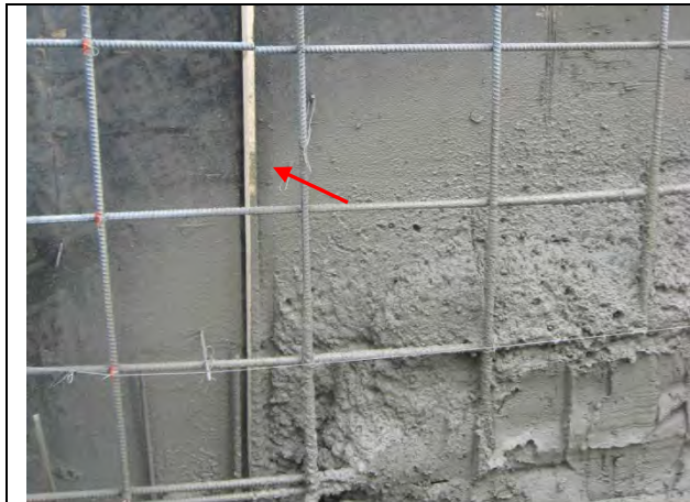
Two-sided forms with wooden strip on receiving surface
