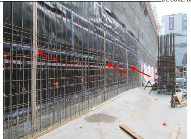
Blind Wall with PVC on receiving surface
