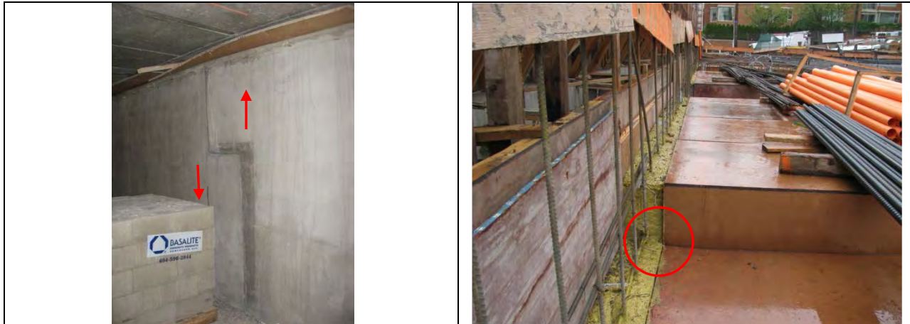
Use control joints to contain cracks that propagate from corners.
