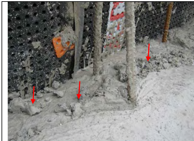
Hammer out protrusions before installing Krystol Waterstop Treatment
