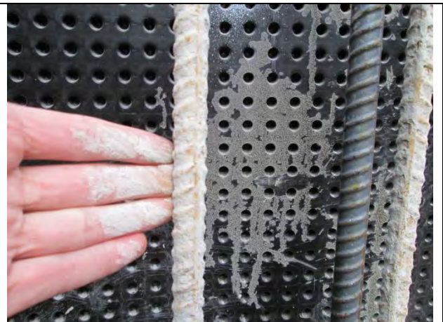
Remove dirt and contaminates from reinforcement
