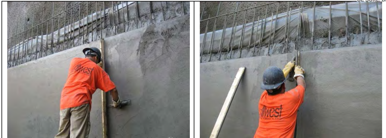
Formation of control joint reveal
