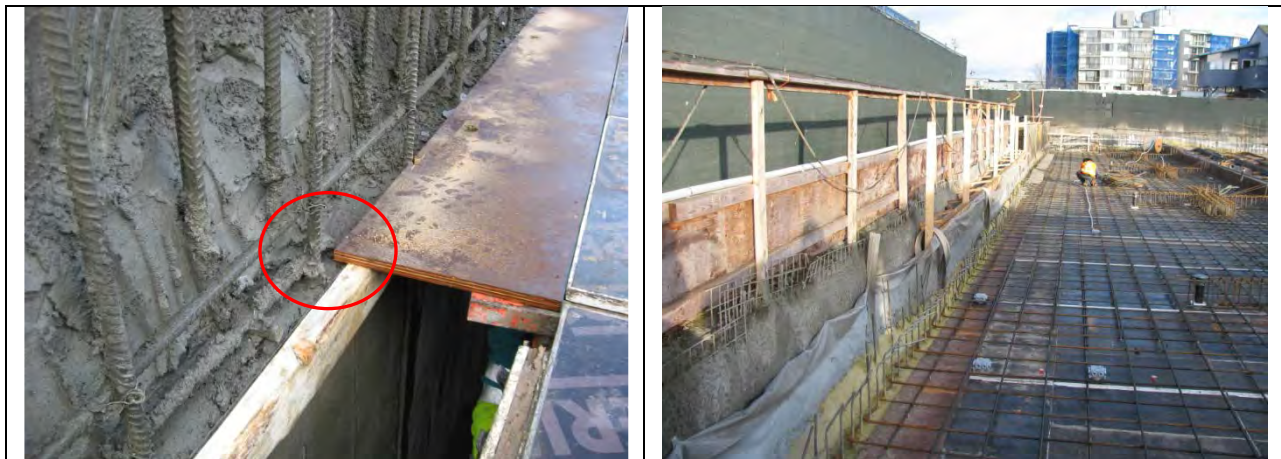
Joint prepared for slab pour (with top-of-wall reveal)
