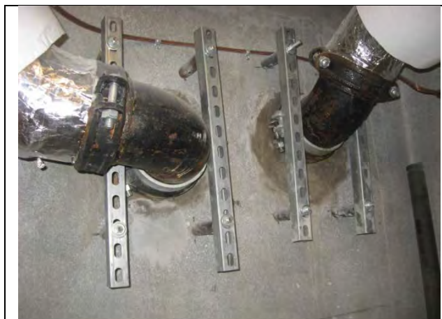
Typical Pipe Penetration
