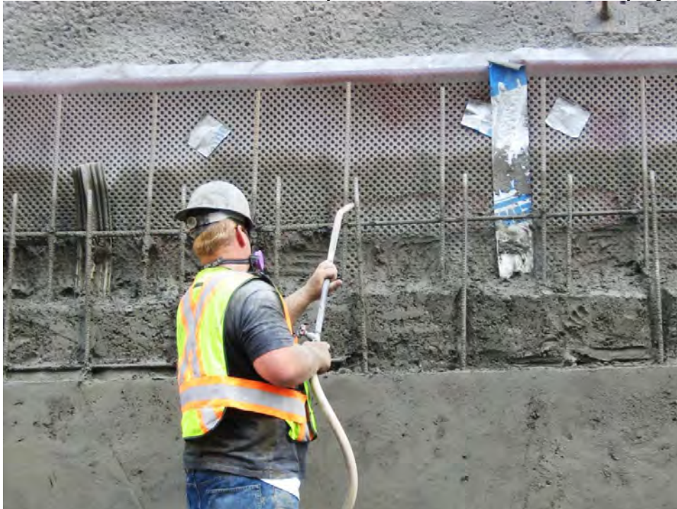
Double check clearance around exposed rebar and remove all overspray
