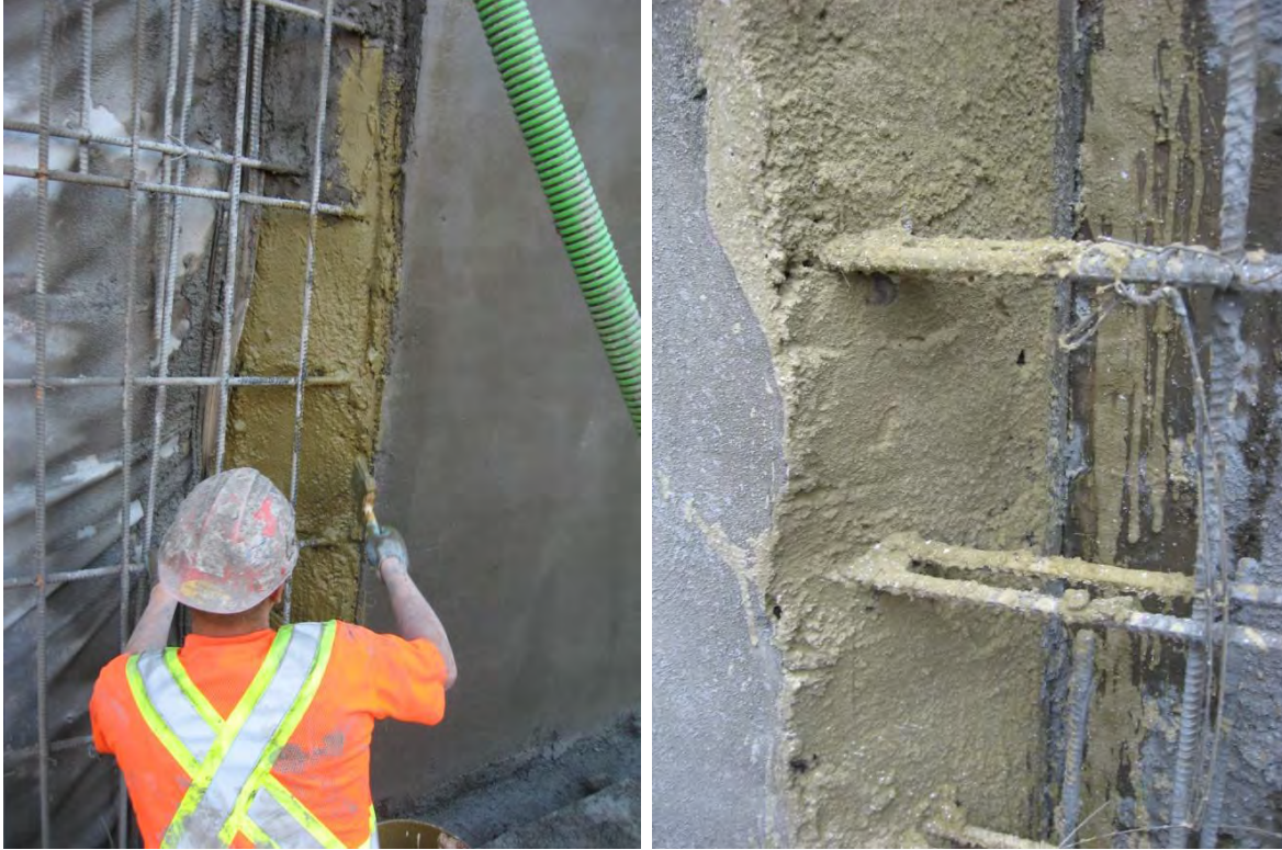
Typical Vertical Wall Joint
