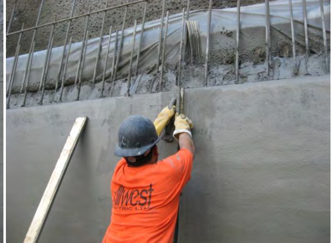
Press keyways into the shotcrete while still plastic
