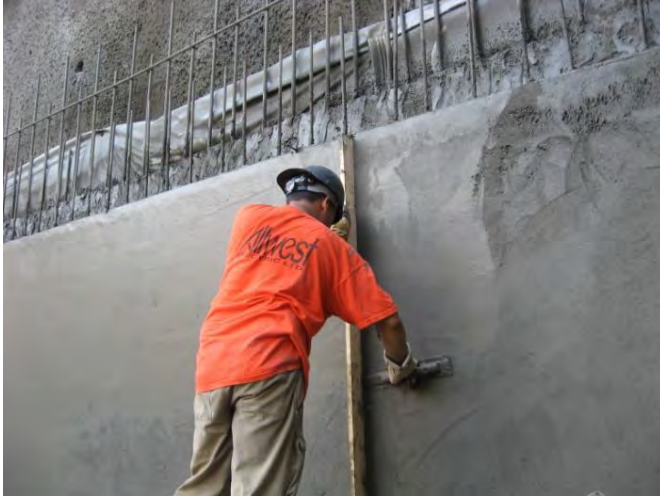
Press keyways into the shotcrete while still plastic
