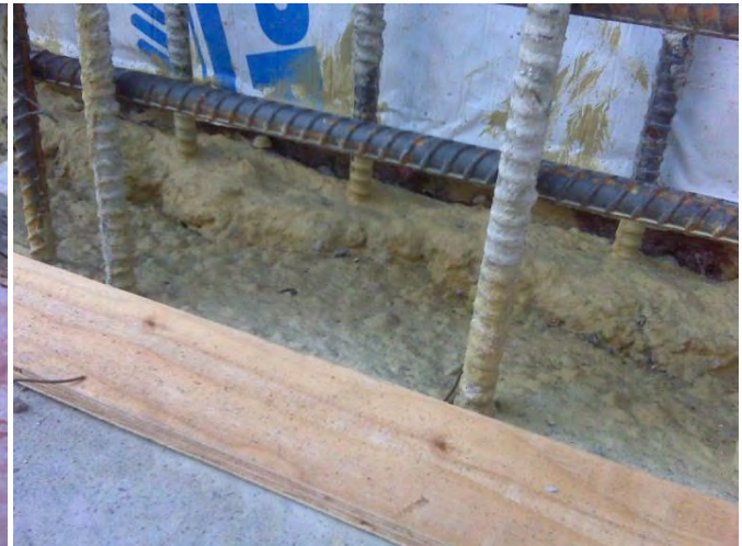
Typical joint after slab pour, ready for the next wall shoot.
