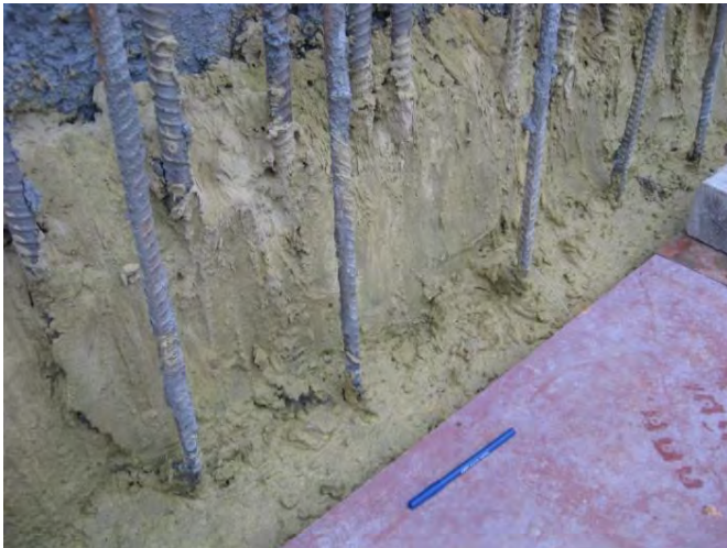
Typical joint with Treatment prior to slab pour
