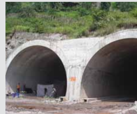
Repair work on the Yunnan Shuima Tunnels
