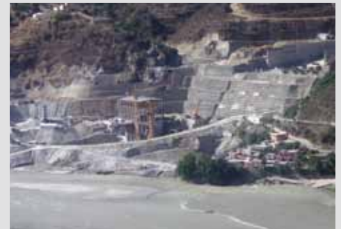
Alakanada Dam, India
