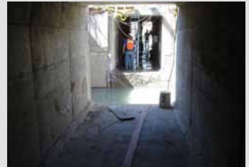
Ensenada International Terminal Tunnel, Ensenada, Mexico
