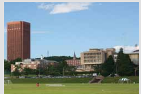
University of Massachusetts Amherst - Boyden Tunnel, USA
