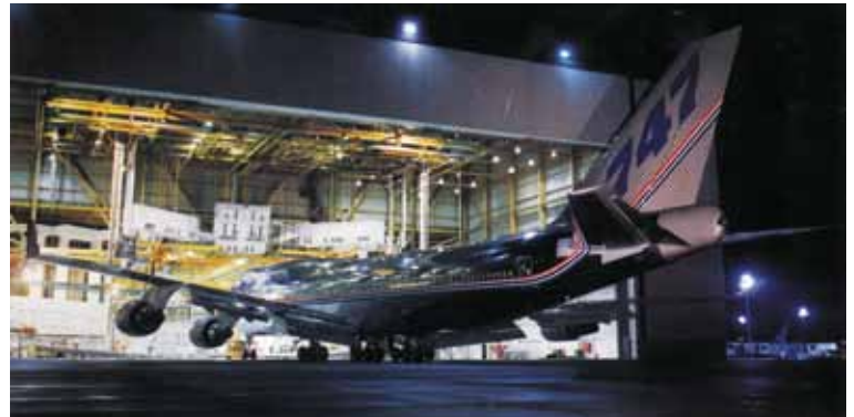
The Boeing Development Center was constructed using KIM in 1983 and has well out lived its warranty.
