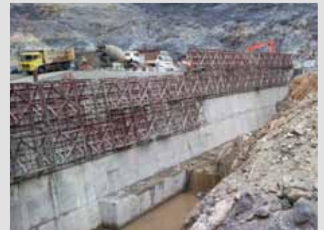
Madushan Dam, Yunnan Province, China
