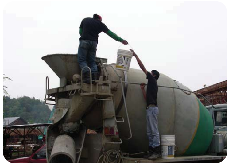
KIM® admixture being poured directly into mixer truck.
