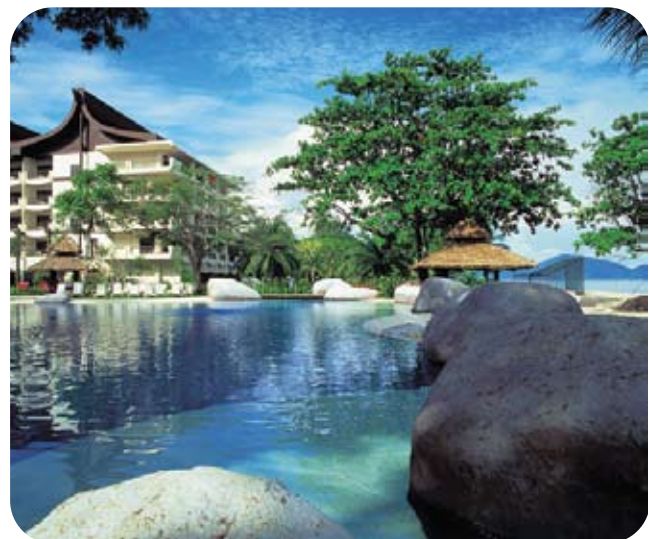
Shangri-La's Rasa Ria Resort poolside rendering when completed. The new swimming pool will be waterproofed with KIM® admixture in all the slabs and Krystol Waterstop System™ for all the joint areas.
