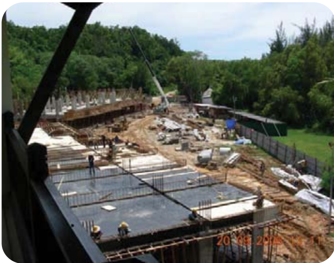
Extension of 2 Blocks of Hotel Rooms (90 rooms) in progress.
