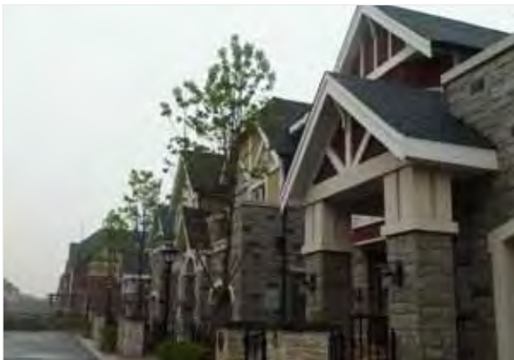
Finished homes at the Vancouver Forest Development in China.
