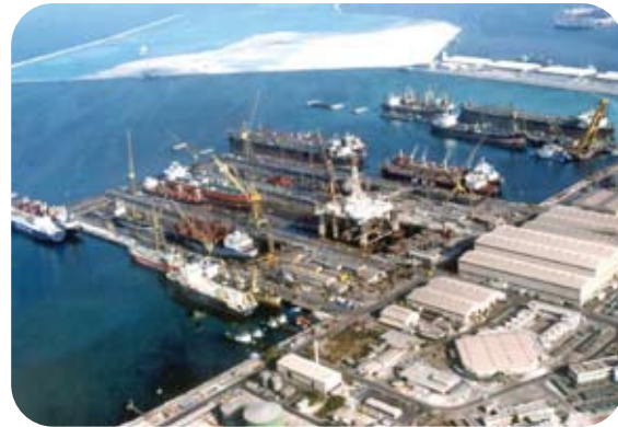
Dubai drydocks aerial view
