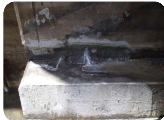
Crack repair as of June 8, 2006
